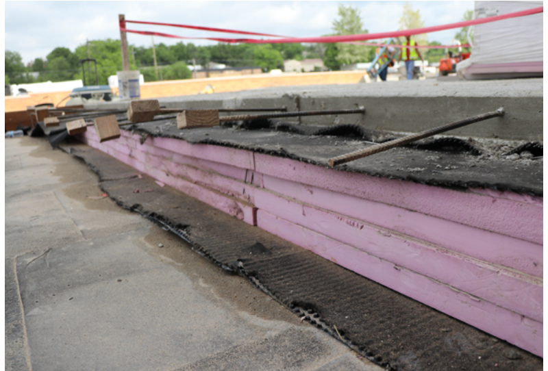
Above: Three layers of FOAMULAR® XPS Insulation deliver compressive strength to withstand traffic on the plaza deck covering 140,000 square feet.
