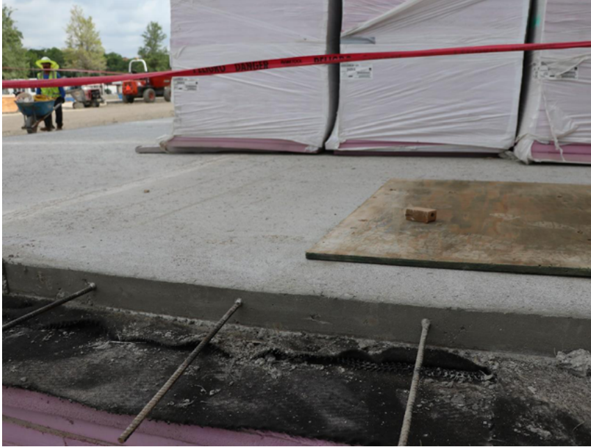
Above: Materials used in the plaza deck were carefully staged on the job site and protected from the elements. The material was installed in phases. Here, the edge of a completed phase shows the layers of XPS, drainboard, and reinforced concrete topping slab ready for transition to the next phase.
