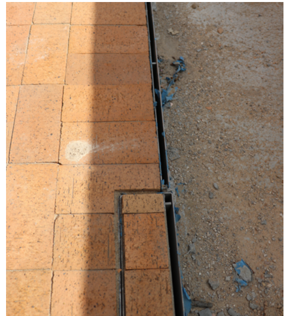
Above: Linear trench drains serve as an efficient open joint to efficiently distribute heavy surface water to sewer lines without disrupting the smooth aesthetic of the deck.
