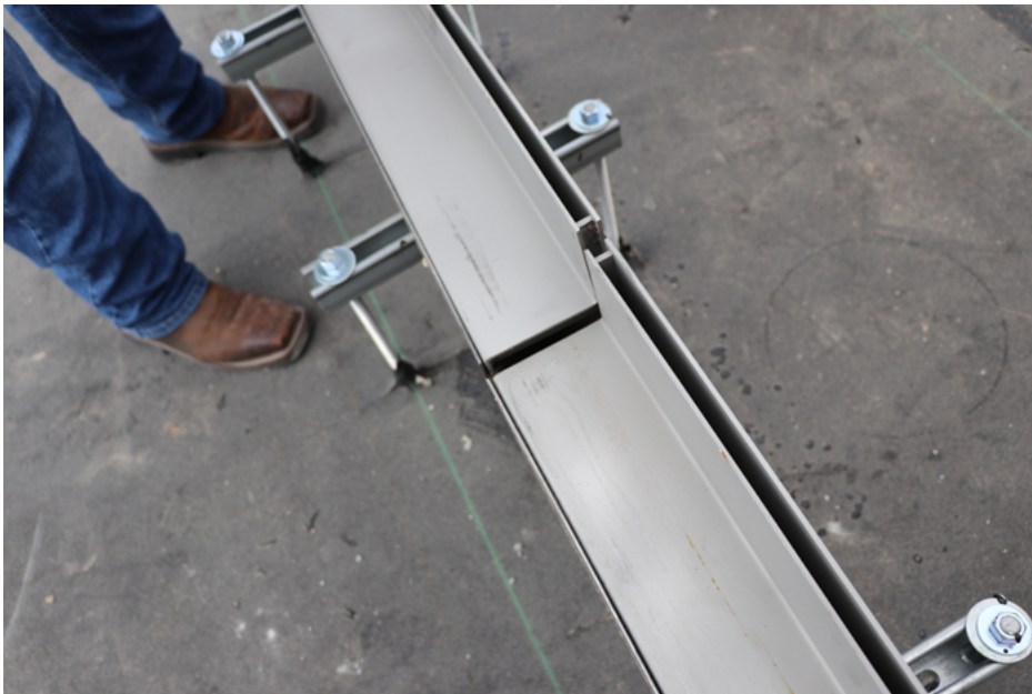
Above: Linear trench drains serve as an efficient open joint to efficiently distribute heavy surface water to sewer lines without disrupting the smooth aesthetic of the deck.
