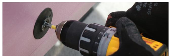
4. Fastener spacing shall be evenly distributed and the minimum necessary per job site conditions as required by Insulation & Fastener Manufacturers to hold the continuous insulation in place until cladding attachment system can be installed to permanently secure the insulation board.
