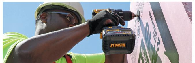
3. Drive fasteners so the washer is tight and flush with insulation surface but do not countersink.
