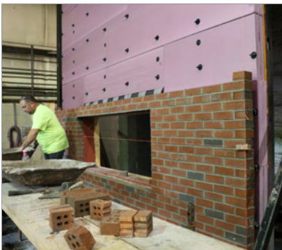
Figure 3: FOAMULAR® NGX™ test wall under construction
