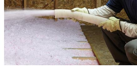
AttiCat® PINK® Blown-In Insulation is a loosefill Fiberglas™ thermal insulation. It is designed for use exclusively with the AttiCat® machine.
