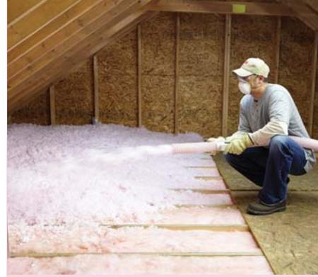
**AttiCat® Expanding Blown-in Insulation Machine breaks up and conditions the AttiCat® Expanding Blown-in PINK® Fiberglas™ Insulation throughout the length of the hose to increase insulating power.**
