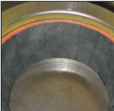
Figure 29 - View of insulation inside reducer
