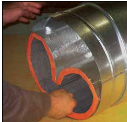
Figure 16 - Inserting gore into elbows
