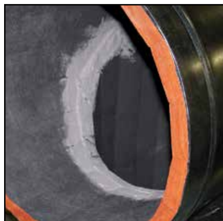
Figure 22 - Coating on the inside edge of Tee
