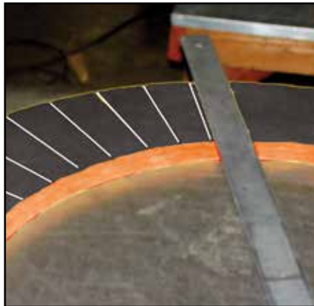
Figure 26 - Marking out groove lines
