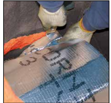
Figure 20 - Trimming straight leg of Tee
