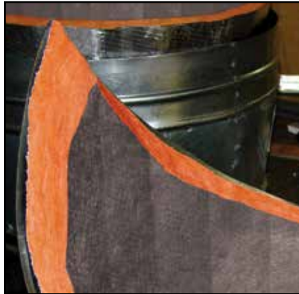
Figure 19 - Trimmed branch leg of Tee
