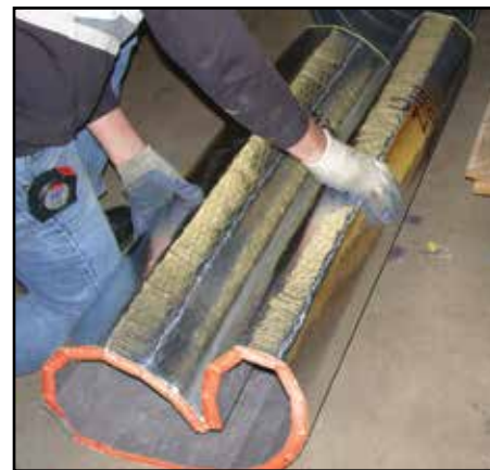
Figure 10 - Heart shape for insertion into duct
