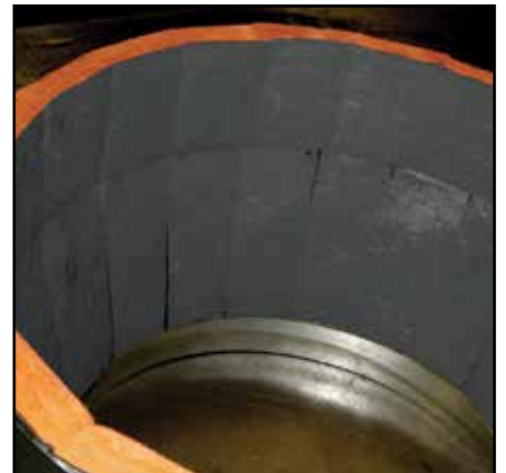
Figure 30 - View of reducer insulation to flange insulation
