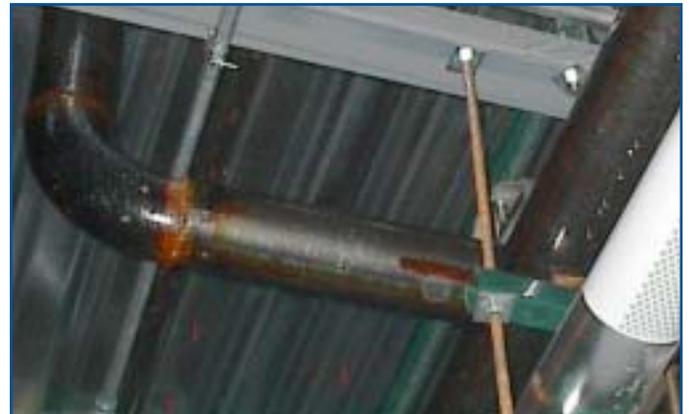
Dripping pipe presented a serious problem for Justen because specifications for chilled water systems require standard insulation to be installed on pipe that is dry and clean.
