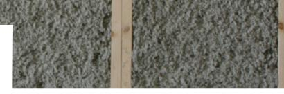
Thermafiber® INSUL-FILL® side wall spray mineral wool insulation is a specially formulated insulation that can be combined with a separate water/latex adhesive solution at the point of insertion to provide:
