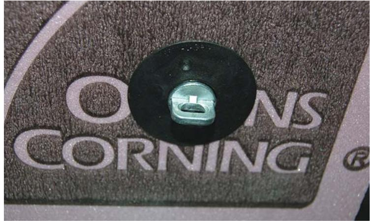
Pos-I-Tie® Barrel screw and Rodenhouse Thermal-Grip® washer
