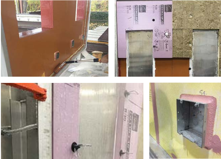
Photos: Penetrated wall under construction and during water resistance testing
