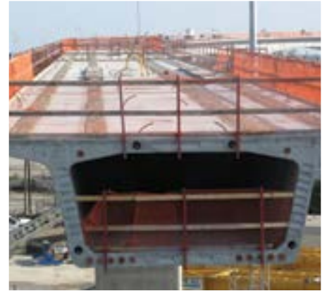
Miami Metro Rail – Deck Bars for electrical isolation in Segmental Precast
