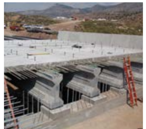
Utah DOT – Emma Park Bridge Precast Deck Panels
