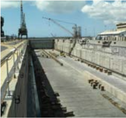
Dry dock – Marine structures
