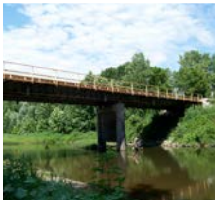
Missouri DOT – Boone Co Bridge
