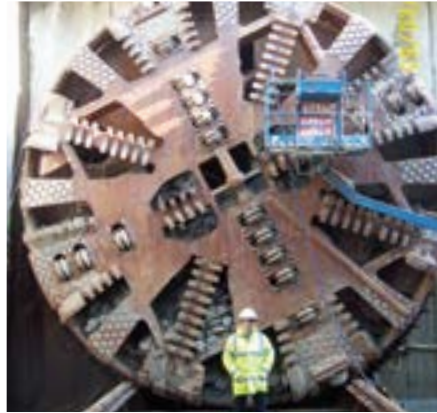
Channel Tunnel TBM – Tunneling
