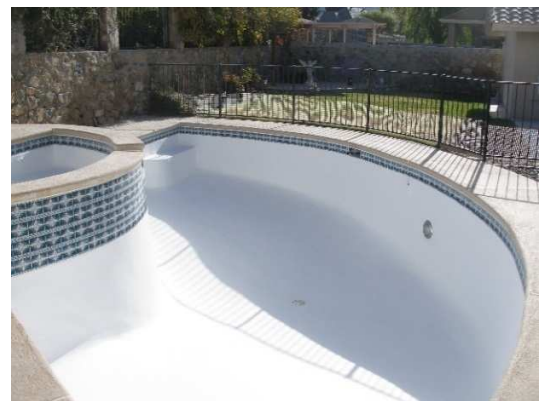
Figure 2 Resurfaced concrete pool with FRP finish
