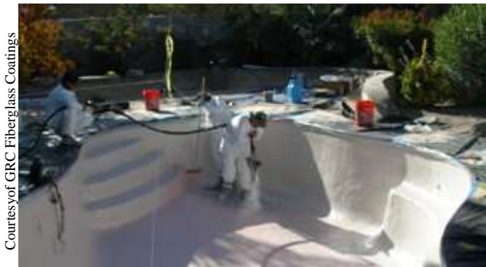
Figure 1 Applicators applying OptiSpray™ H roving to the interior of a swimming pool
