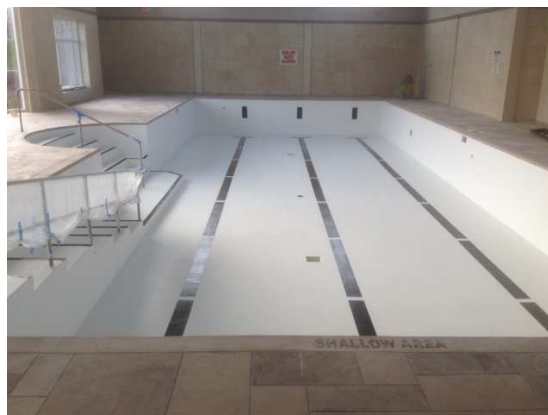
Figure 3 Commercial pool finished with FRP lining incorporating OptiSpray™ H roving
