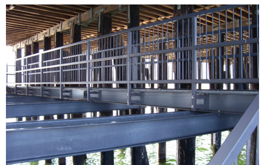
Picture courtesy Strongwell, USA (under a bridge)
