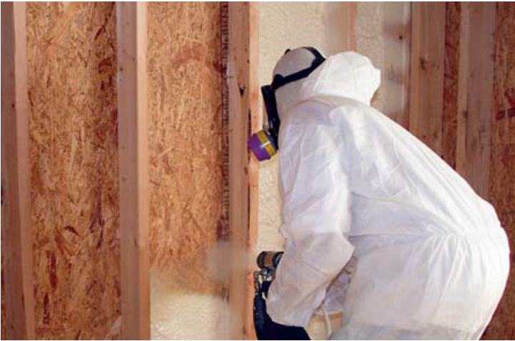
NIOSH recommends that SPF installers wear extensive personal protective equipment including full-face supplied-air respirators and chemical protective clothing during installation. 1 The home must be quarantined for up to 72 hrs. 3
