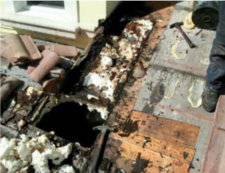
OSB and plywood manufacturers, as well as the Engineered Wood Association, are beginning to provide recommendations to avoid the use of SPF under roof decks due to rot. (Photo credit: The Florida Roofing, Sheet Metal, and Air Conditioning Contractors Association)
