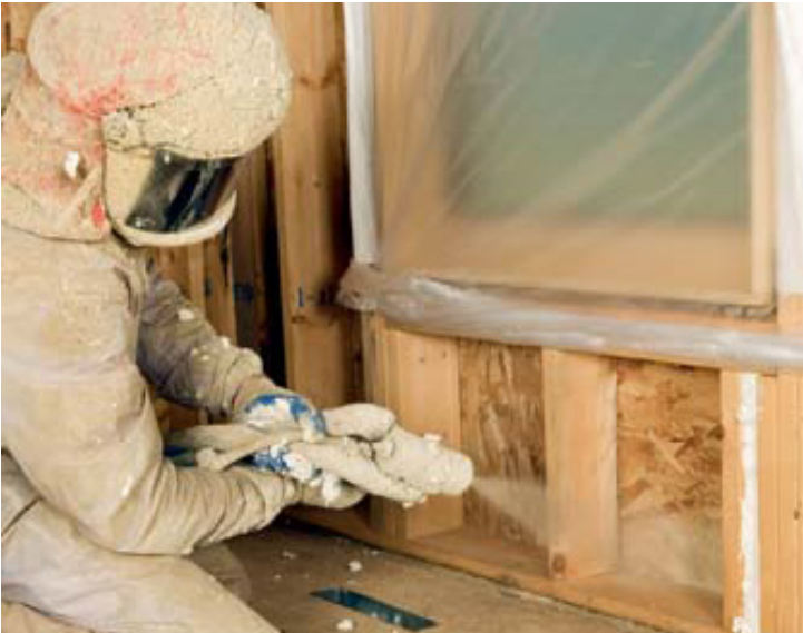
SPF installers must wear extensive personal protective equipment and be fully trained.
