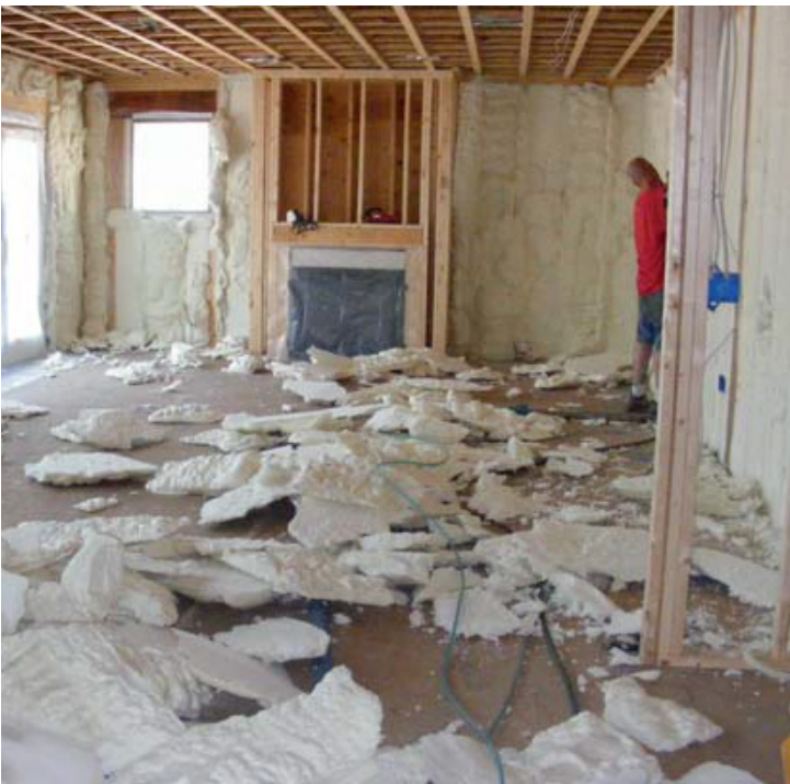
Approximately one-fifth of the material used in a typical open cell SPF job is waste that goes to a landfill. 2
