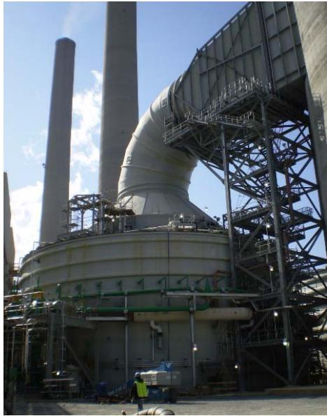
Wet scrubbers remove vast quantities of sulfur dioxide ( $\text{SO}_2$ ) from the exhaust of coal-fired power plants by mixing the flue gasses with water and limestone. They house an unrelenting combination of sandstorm and acid-laced tsunami.
