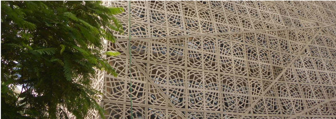
Panels were installed without the need for heavy lifting equipment.
