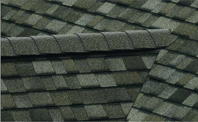
roofing and asphalt
