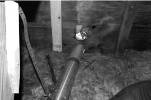
Notice how mold is starting to grow on the underside of the roof deck
